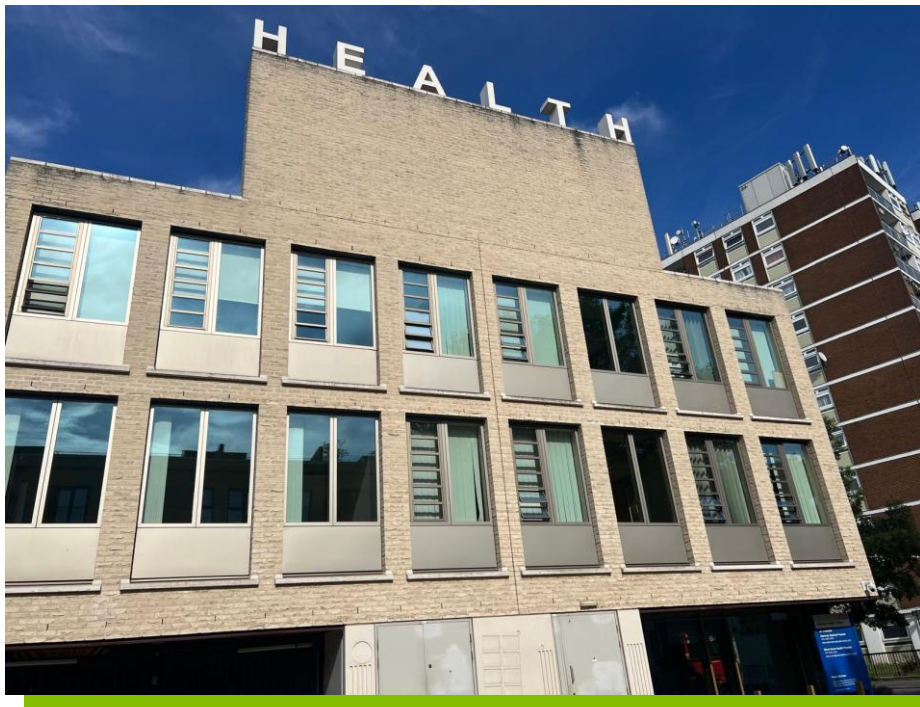
Exterior of Akerman Health Centre.
